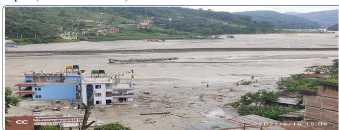
Figure 6.2: Damage due to flood and land slide (2021) on Melamchi bazar and Agriculture land of Sindhupalchok (DODM)
